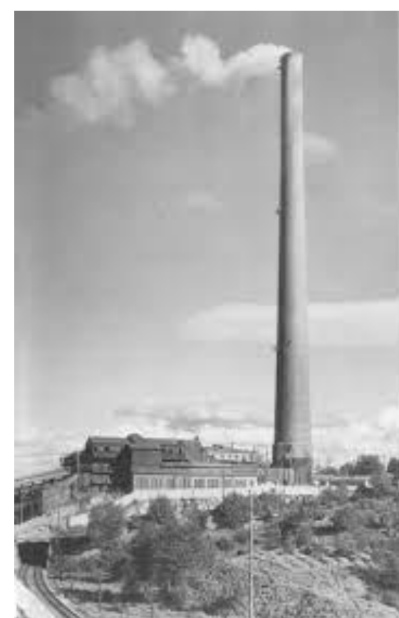
Figure 1. ASARCO co. in Tacoma WA
