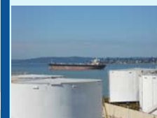
Figure 14: Photograph of Commencement Bay, Tacoma WA.
